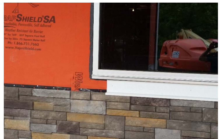
VaproLiqui-Flash (gray) skins-over in 30 minutes and cures in all weather conditions for fast and easy installation.
