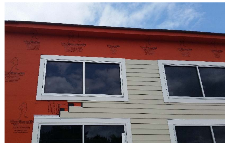
WrapShield SA Self-Adhered has multiple substrate compatibility and is tear, rip and puncture resistant during and after construction.
